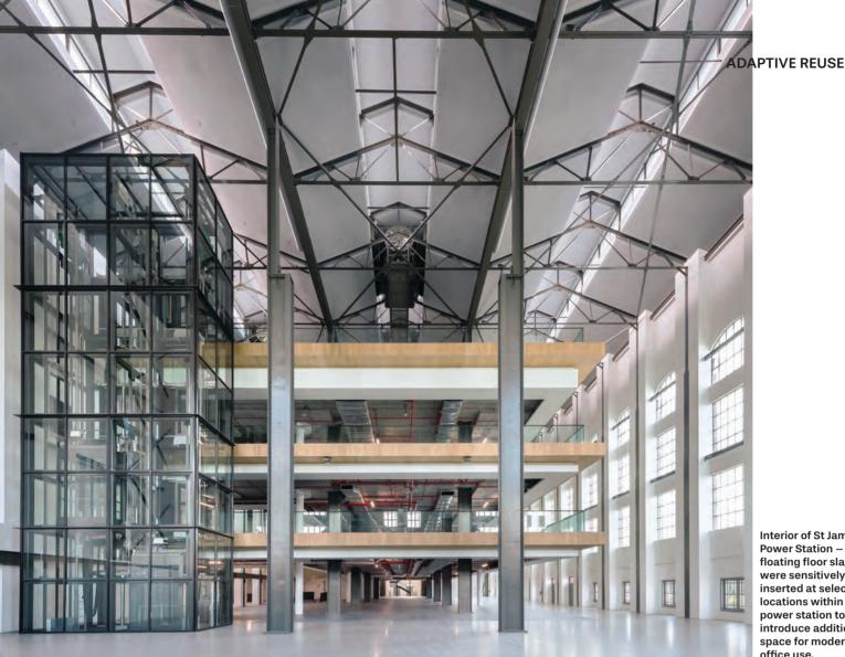
Interior of St James Power Station - New floating floor slabs were sensitively inserted at selected locations within the power station to introduce additional space for modern office use.
