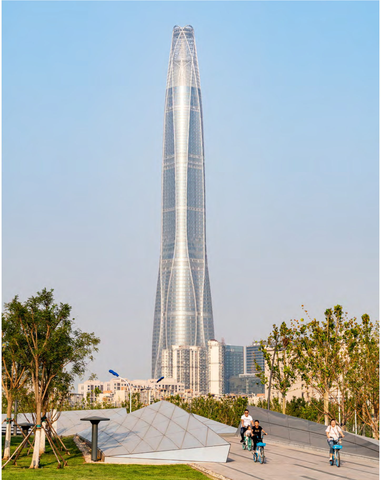
Tianjin Chow Tai Fook Financial Centre. Photography by Seth Powers.
