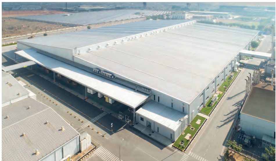
Daikin Factory Ph II in Neemrana, Rajasthan, India. Photo: © Daikin
