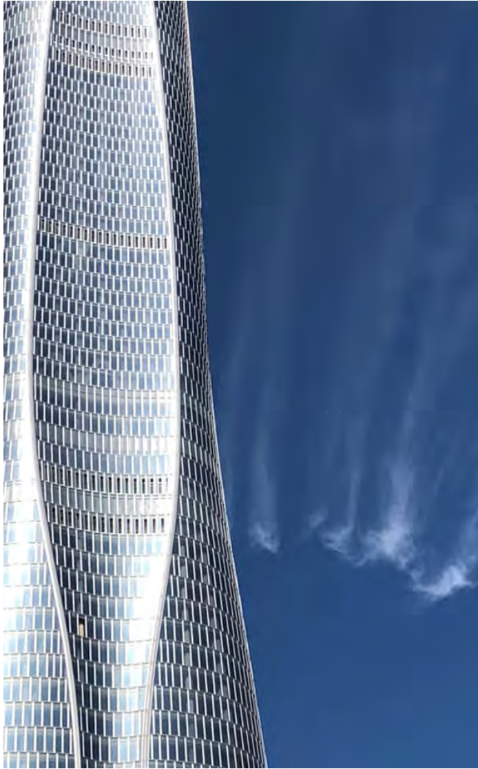
Tianjin Chow Tai Fook Financial Centre façade close-up. Photography by Ronald Lu & Partners.
