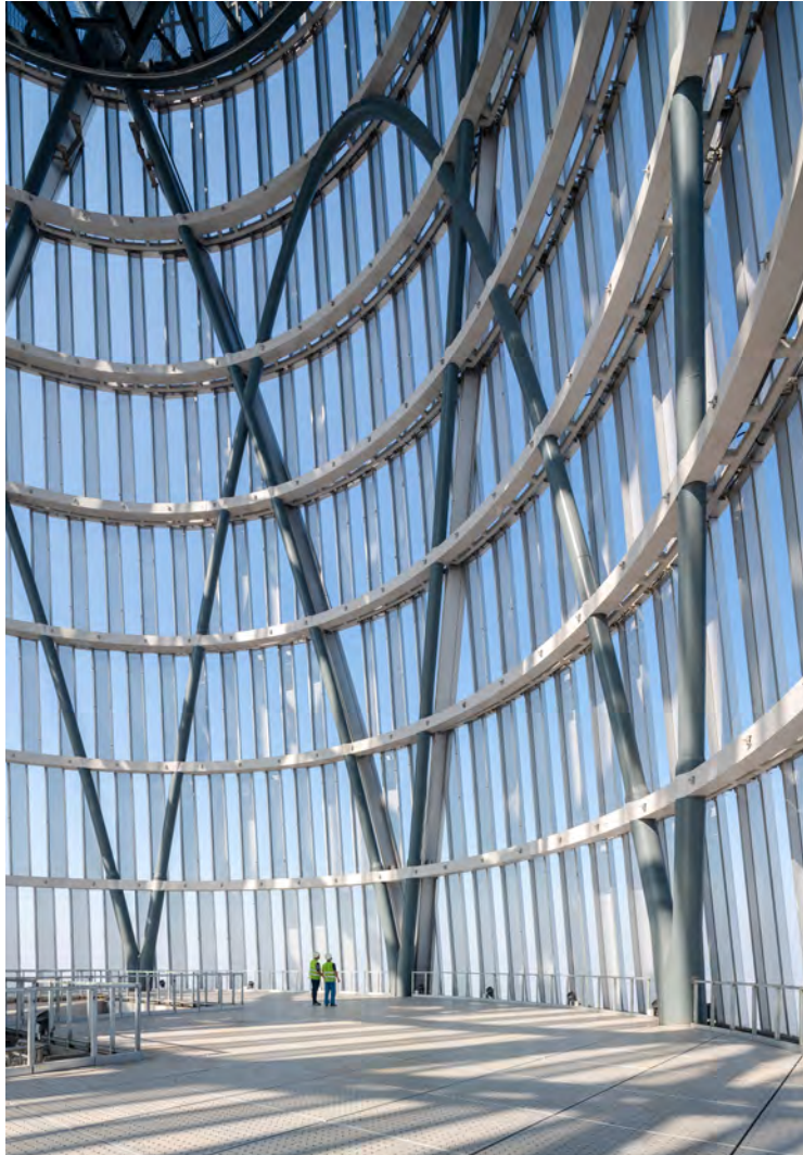
Tianjin Chow Tai Fook Financial Centre. Photography by Seth Powers.
