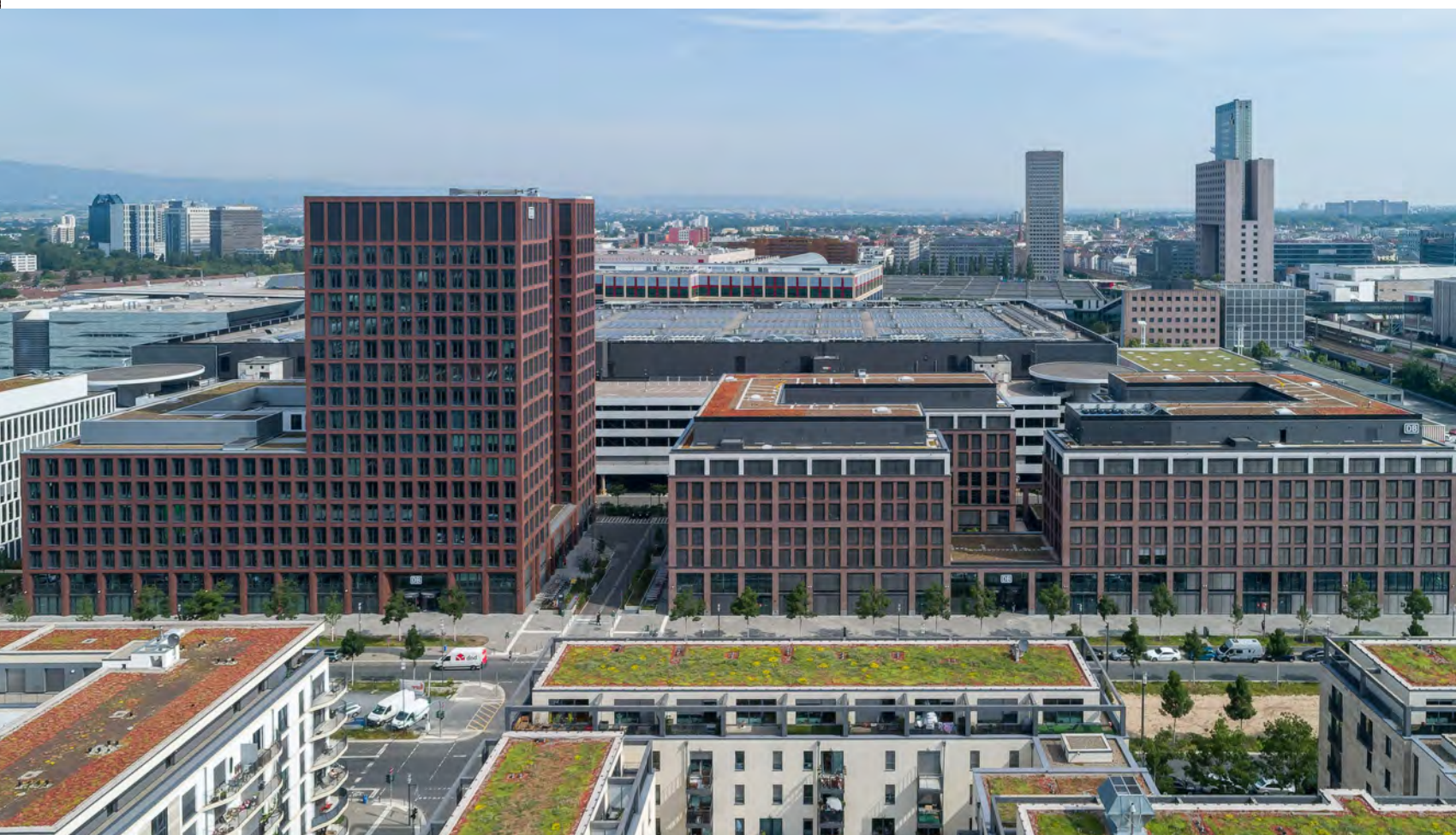
General view of Deutsche Bahn Campus – consisting of DB Brick and Tower along Europa-Allee. © Lars Gruber, Darmstadt
